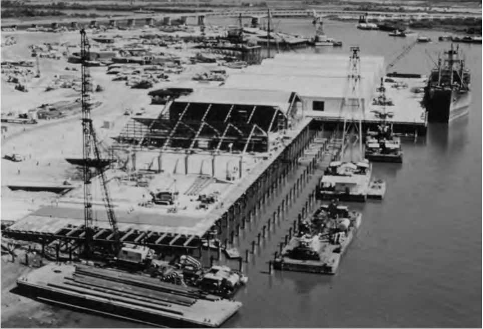
Port and warehouses under construction in late 1966 at Newport
